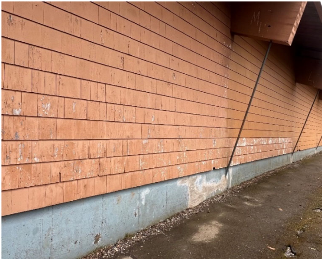
Chipping and Discoloration of Wood Cladding
