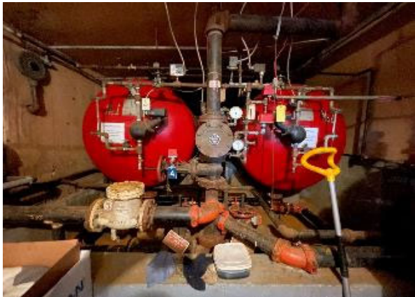
(Top Left) Dry sprinklers serving curling rink. (Bottom Left) Sprinkler tanks and associated piping. (Right) Wet sprinklers serving curling rink observation area.
