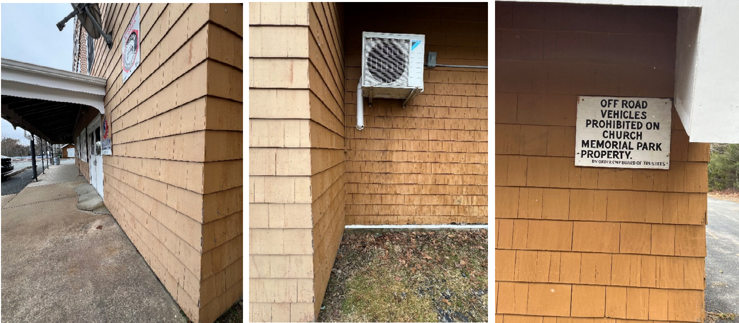
Typical Wood Cladding Condition
