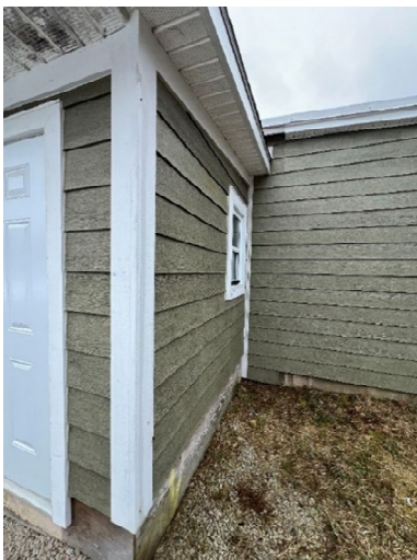
Chipping and Discoloration of Wood Cladding
