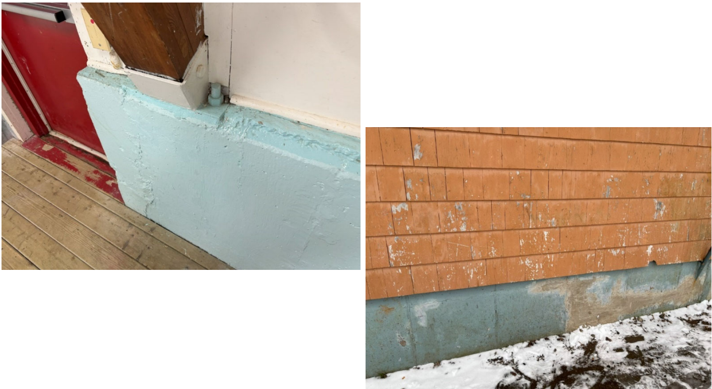
Patched concrete foundation wall on hockey rink exterior & Concrete foundation wall on curling rink interior
