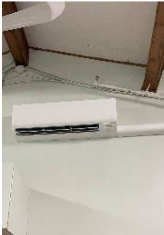
Mini-split heat pumps observed throughout the facility.
