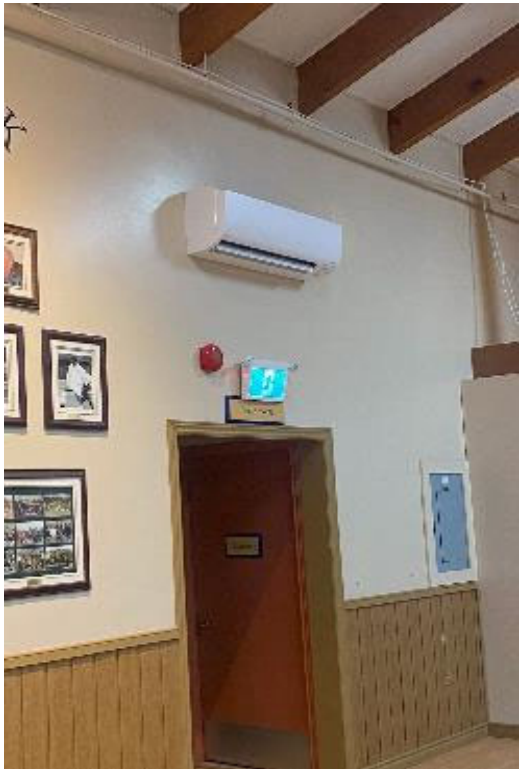
Mini-split heat pumps observed throughout the facility.
