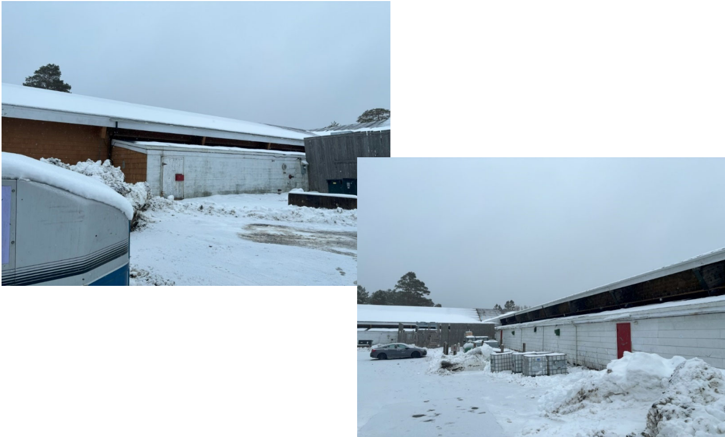
Low roof structure adjacent to curling rink + Low roof structure adjacent to hockey arena
