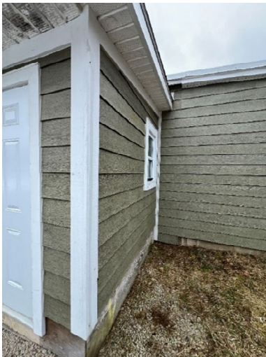
Chipping and Discoloration of Wood Cladding
