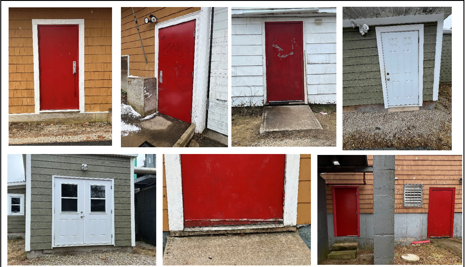
Examples of Other Exterior Doors
