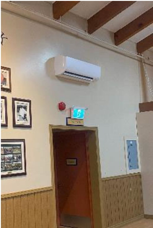
Mini-split heat pumps observed throughout the facility.
