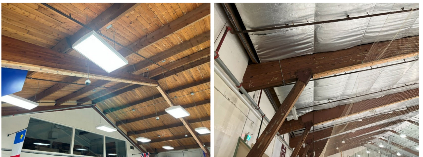
Glulam rafter with completed reinforcing in curling rink & Glulam rafter with completed reinforcing in hockey arena
