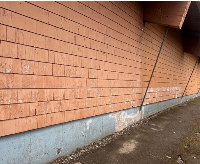
Chipping and Discoloration of Wood Cladding
