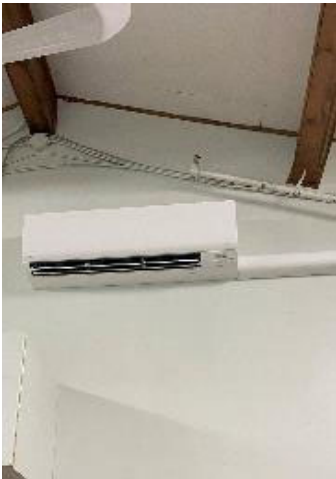
Mini-split heat pumps observed throughout the facility.
